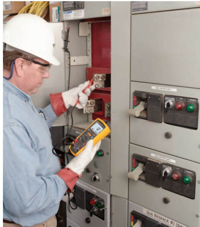
Steve Uhrich tests resistance of drive cabling.
